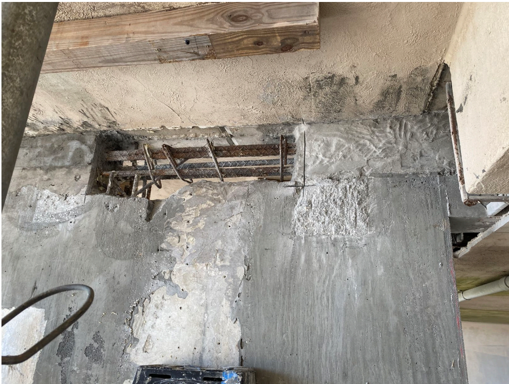
Picture 2: Typical approved concrete repair
