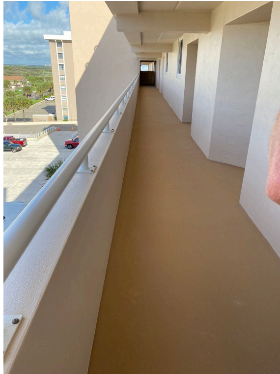
Picture 1: Typical intermediate coat application of walkways
